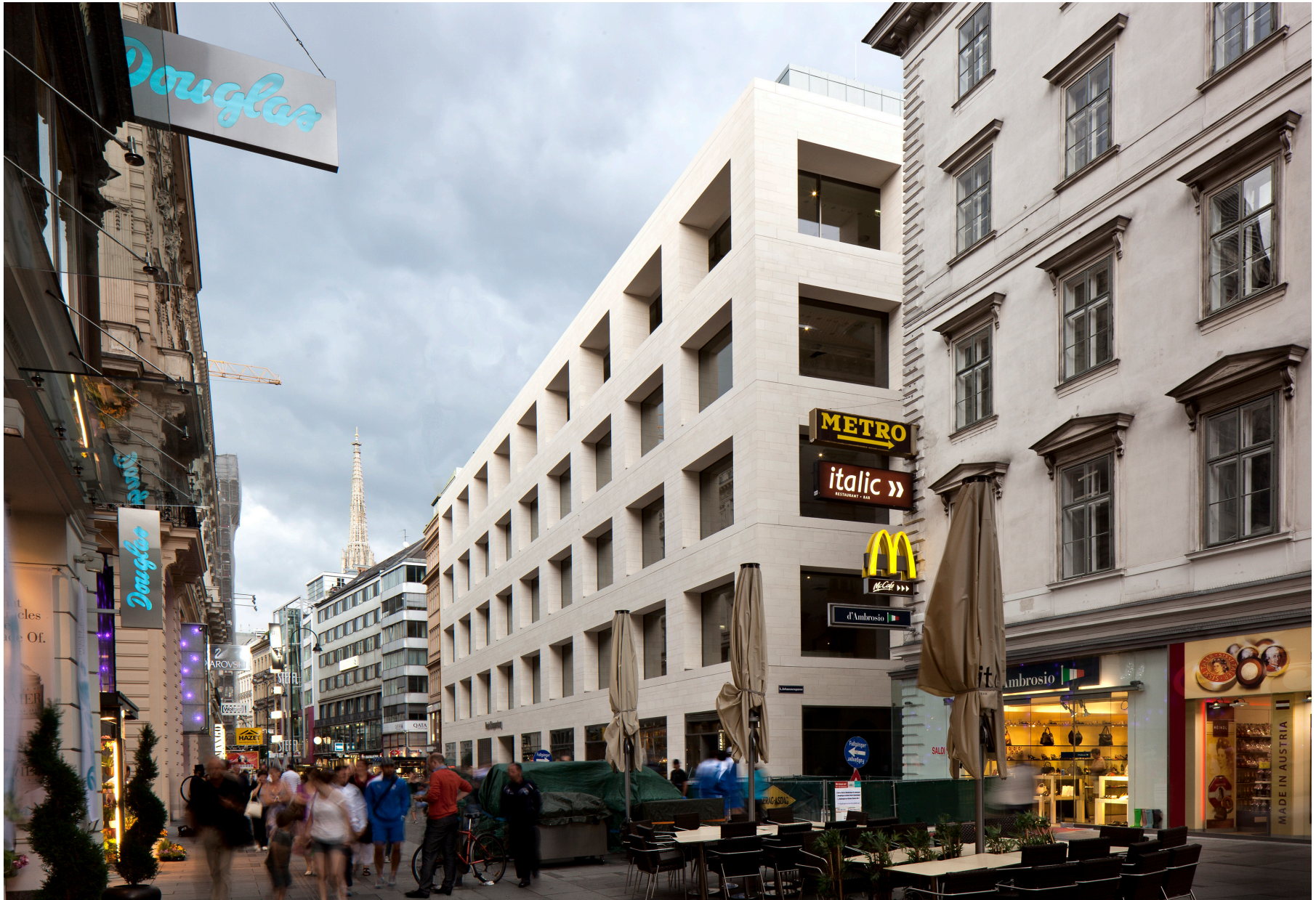
D1 - Boulevard City/ Reference, Peek & Cloppenburg Flagship Store, Vienna, Austria
