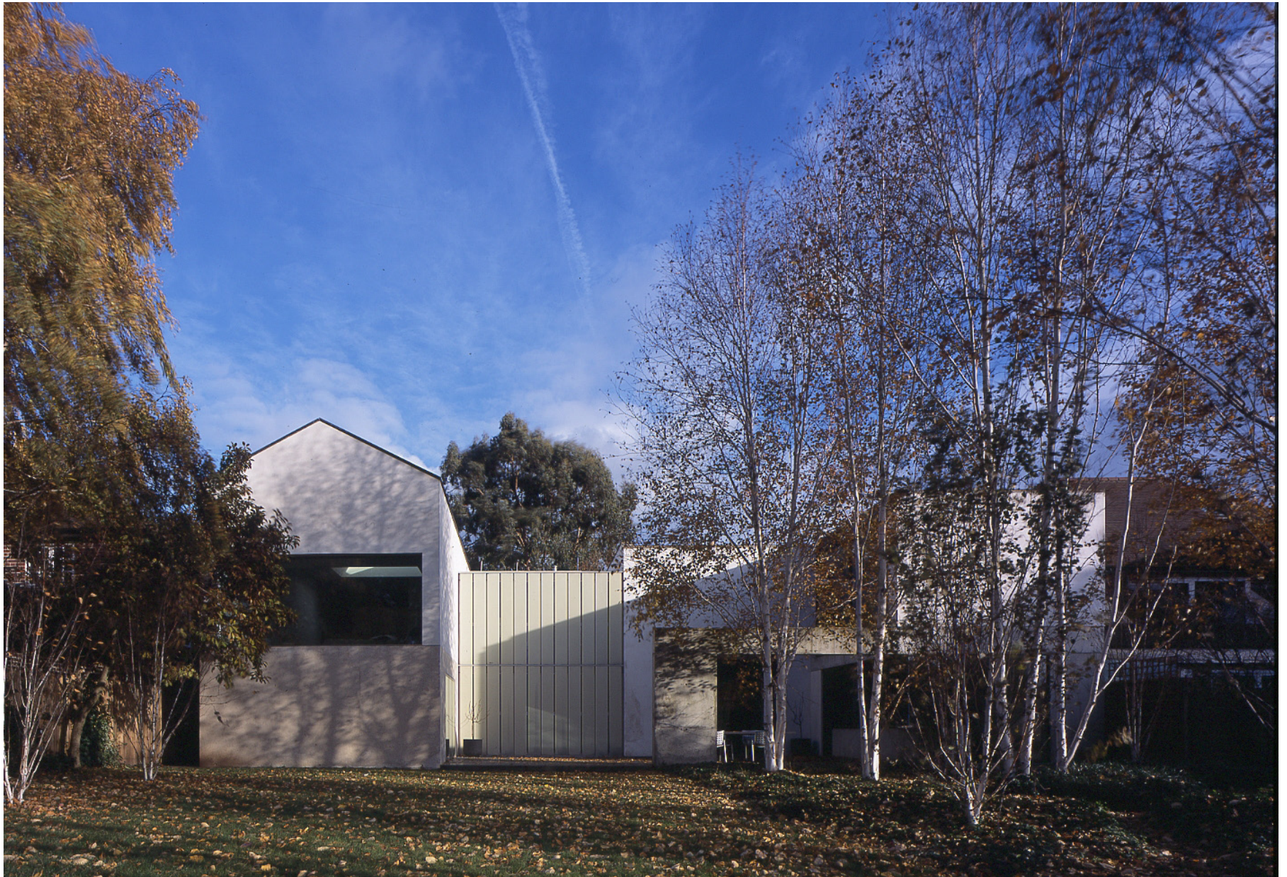
D1 - Family Houses/ Reference, Private House, Richmond, London, United Kingdom
