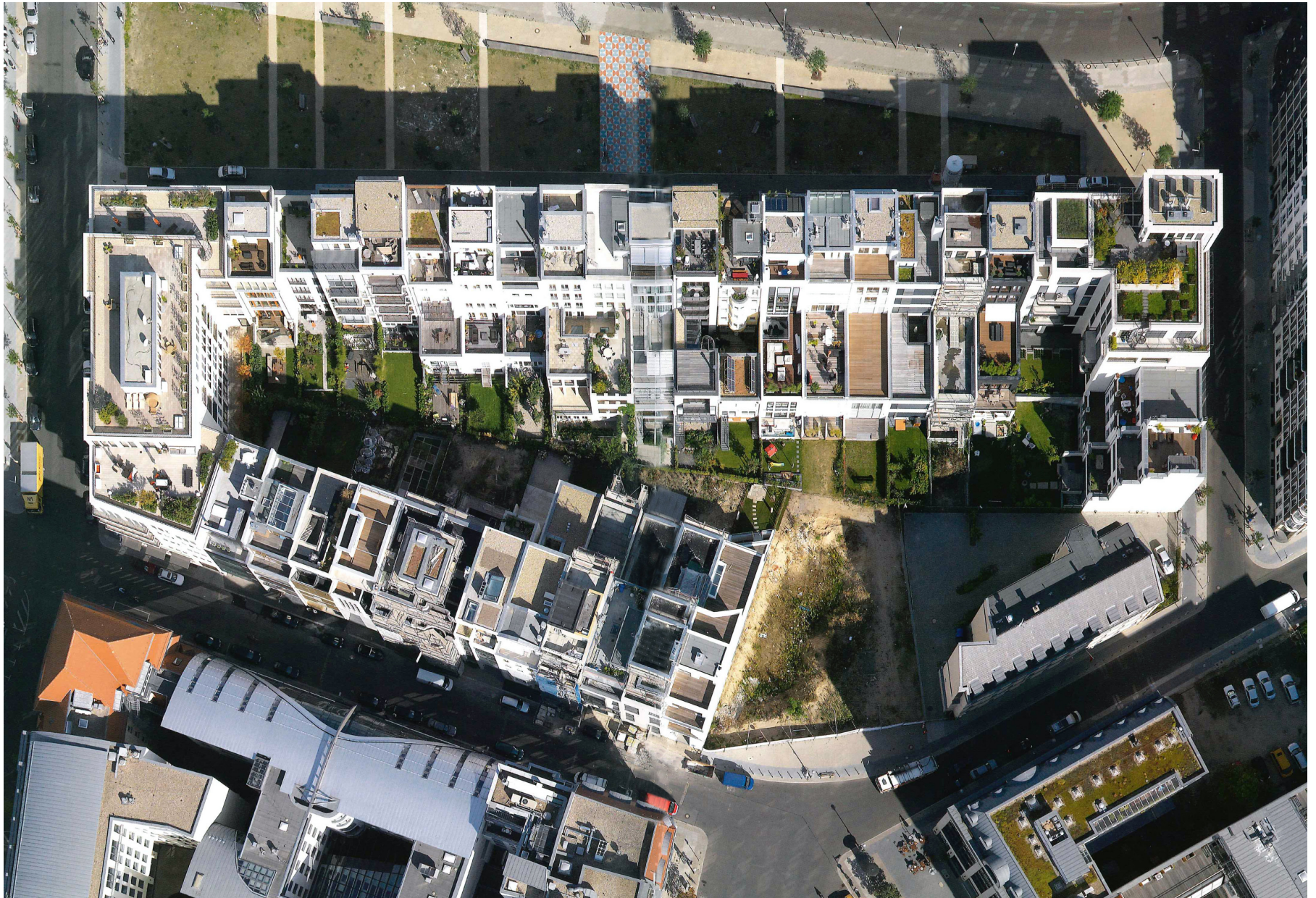
D1 - River Houses/ Reference, Stadthäuser Friedrichswerder, Berlin, Germany
