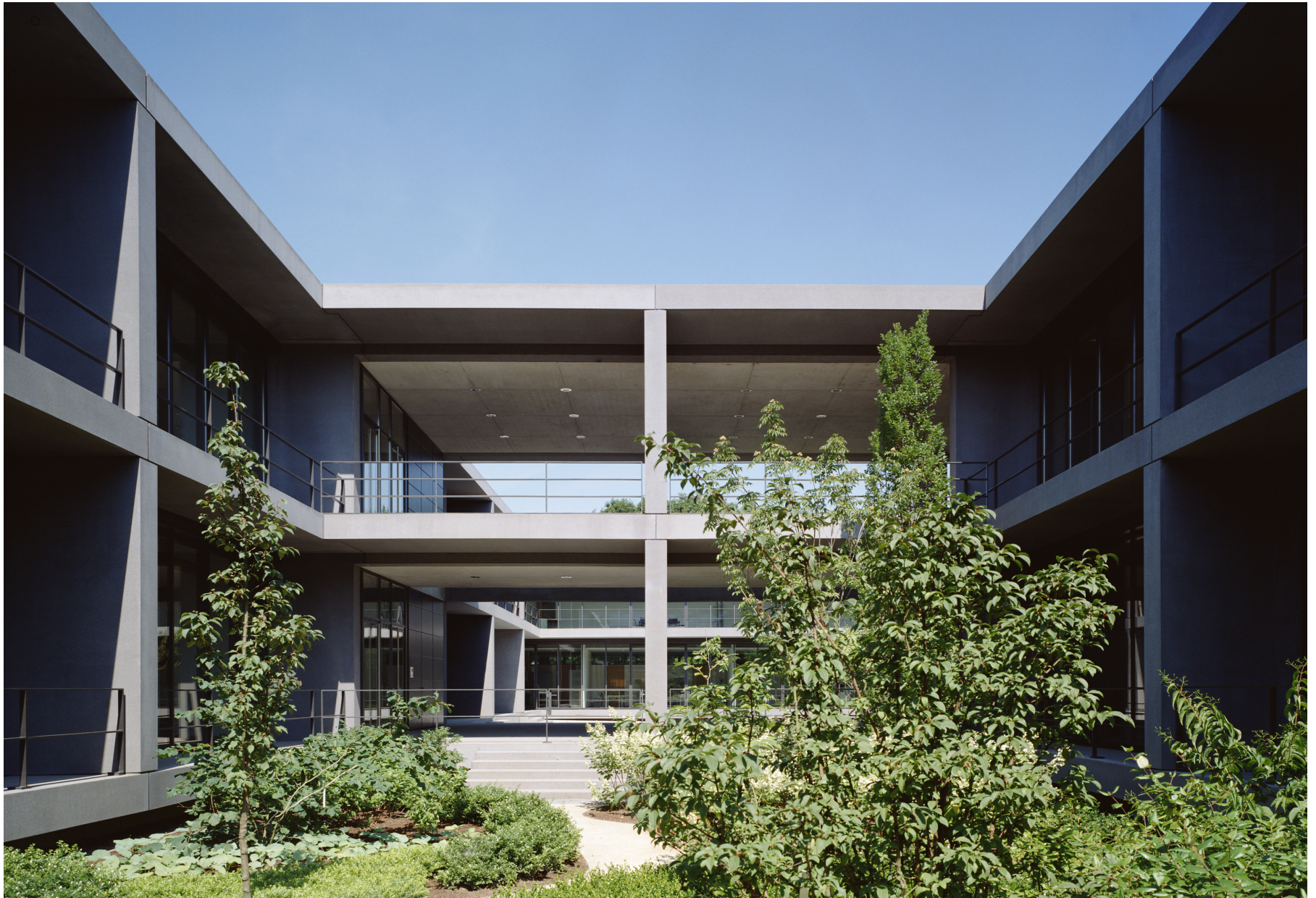
D1 - River Houses/ Reference, Ernsting Service Center, Coesfeld, Germany
